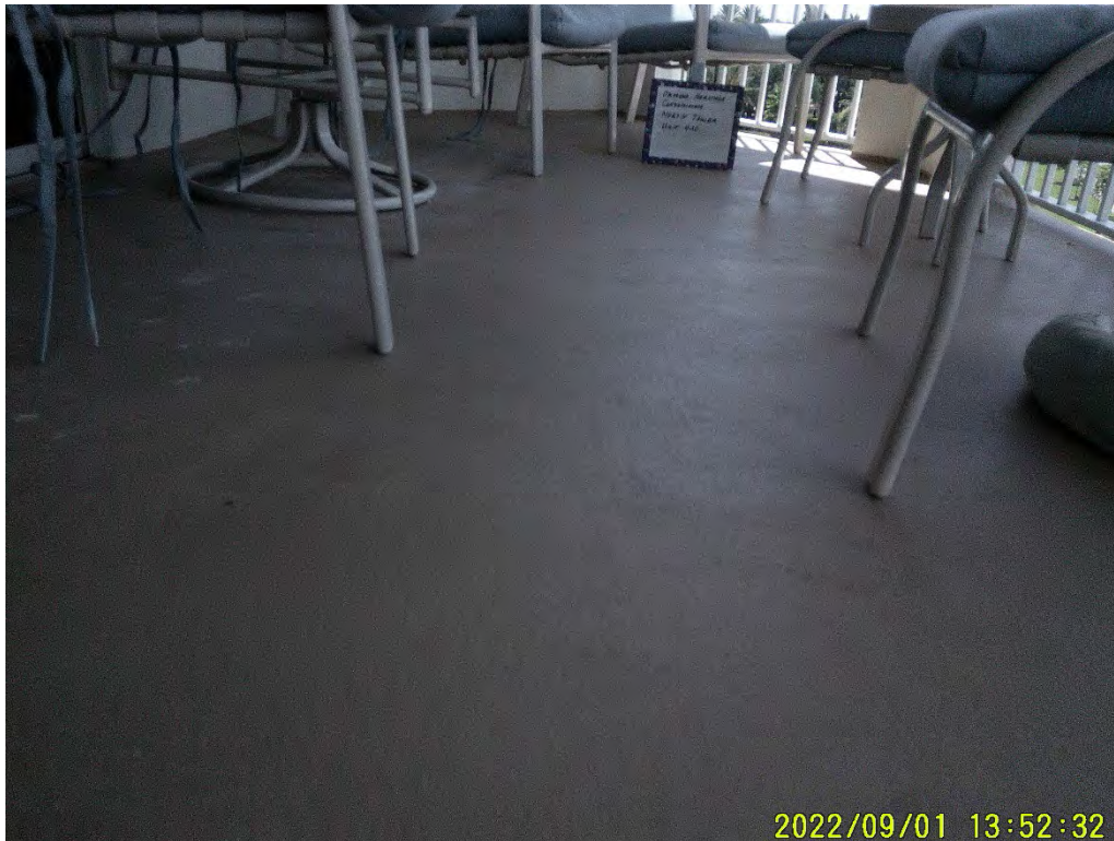
Photograph 57: Balcony (Misc. Location)
