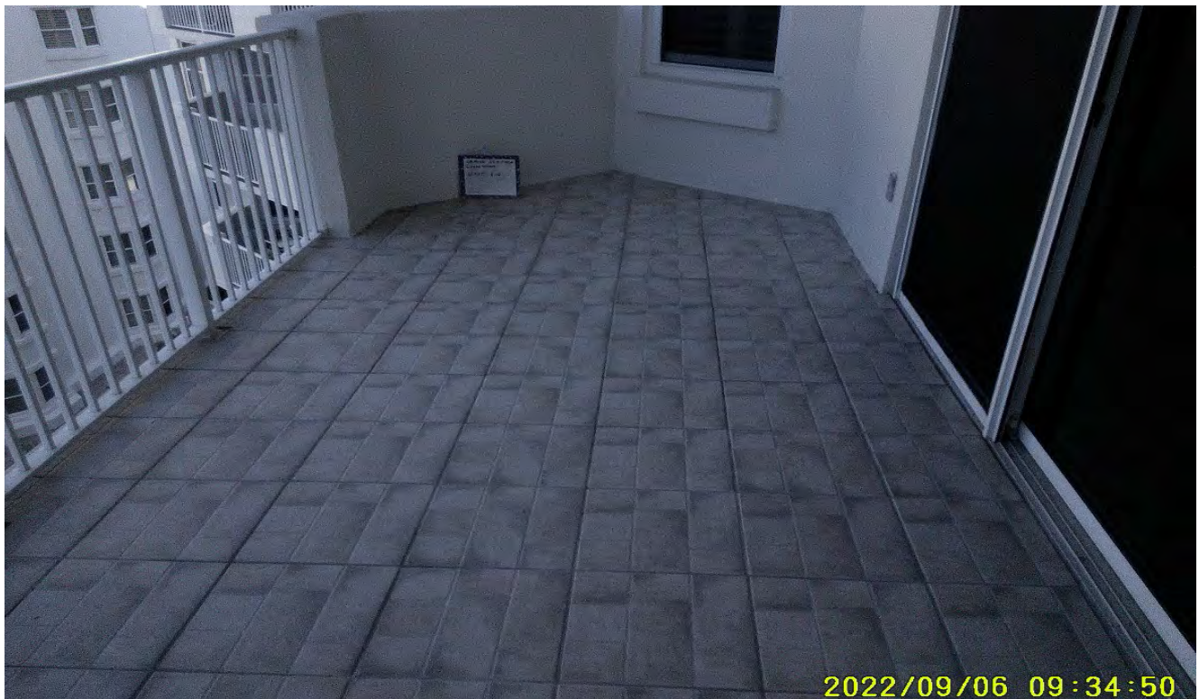
Photograph 2: Balcony (Misc. Location)
