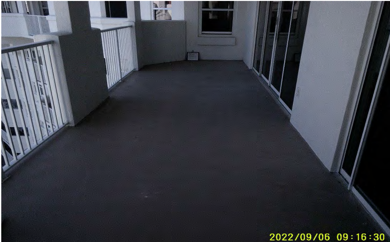
Photograph 11: Balcony (Misc. Location)
