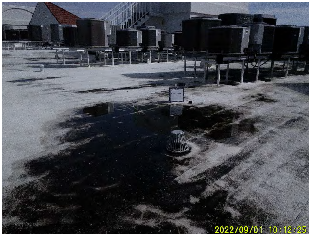
Photograph 86: East Tower, Roof
