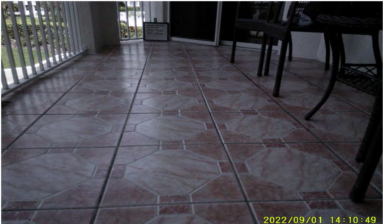
Photograph 53: Balcony, South Tower Unit 204/2
