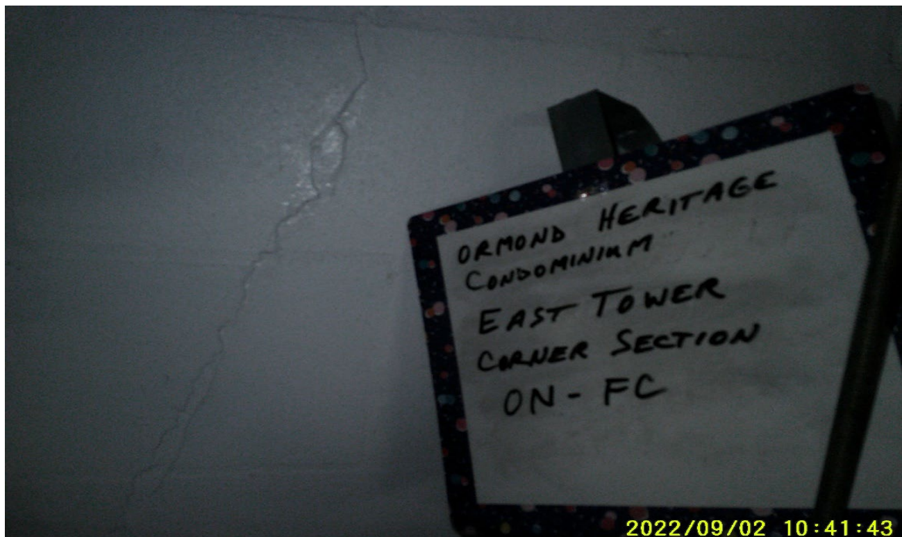
Photograph 22: East Tower, Parking Garage, Section FC
