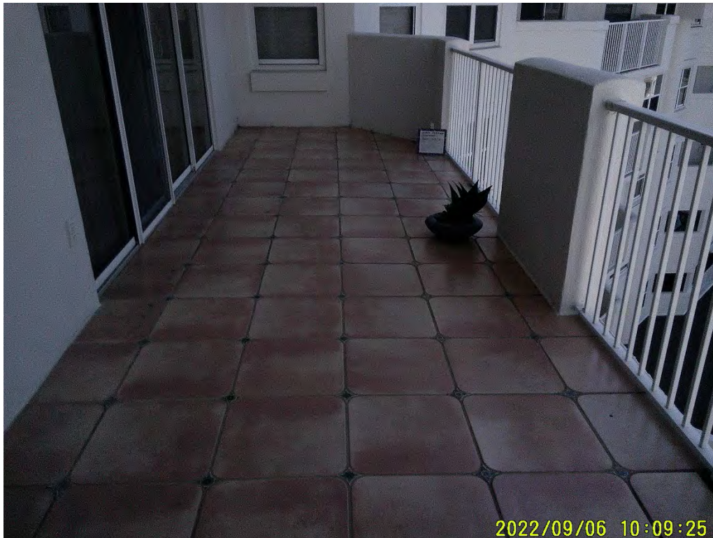
Photograph 95: Balcony (Misc. Location)
