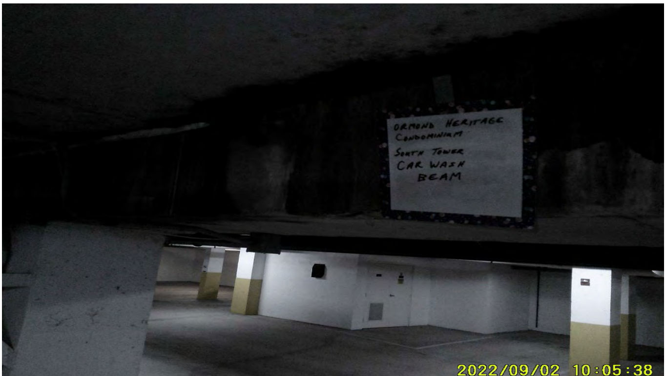
Photograph 32: South Tower, Parking Garage Car Wash
