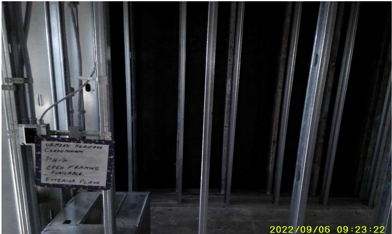
Photograph 7: Phase 2 Open Framing, Ext. Plane
