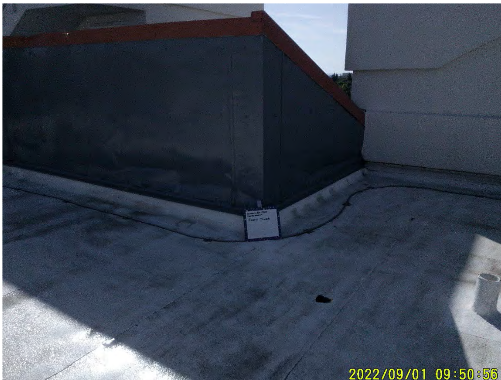
Photograph 90: South Tower, Roof
