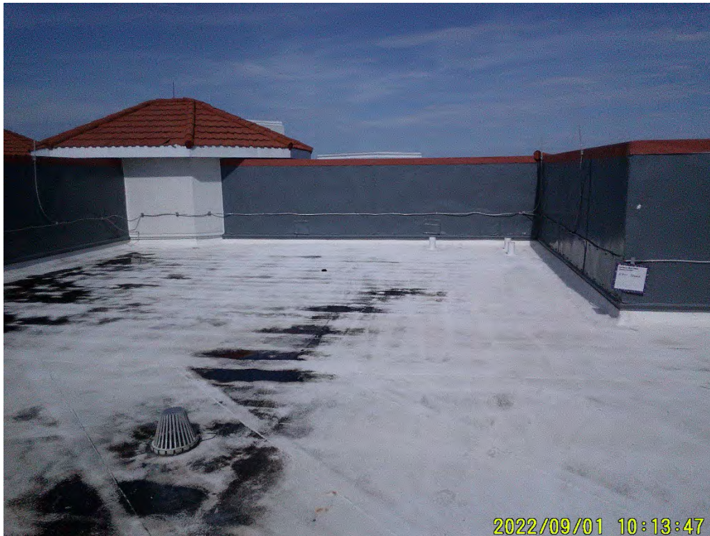
Photograph 85: East Tower Roof
