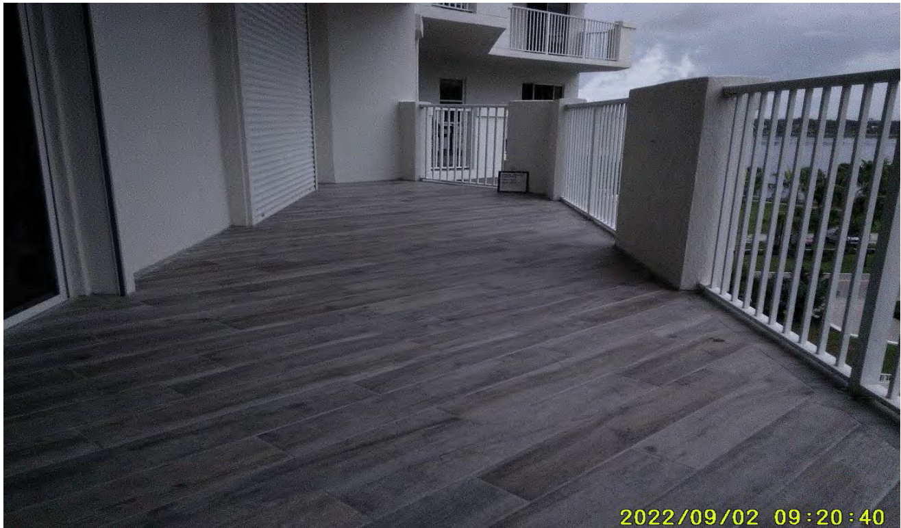
Photograph 43: Balcony (Misc. Location)
