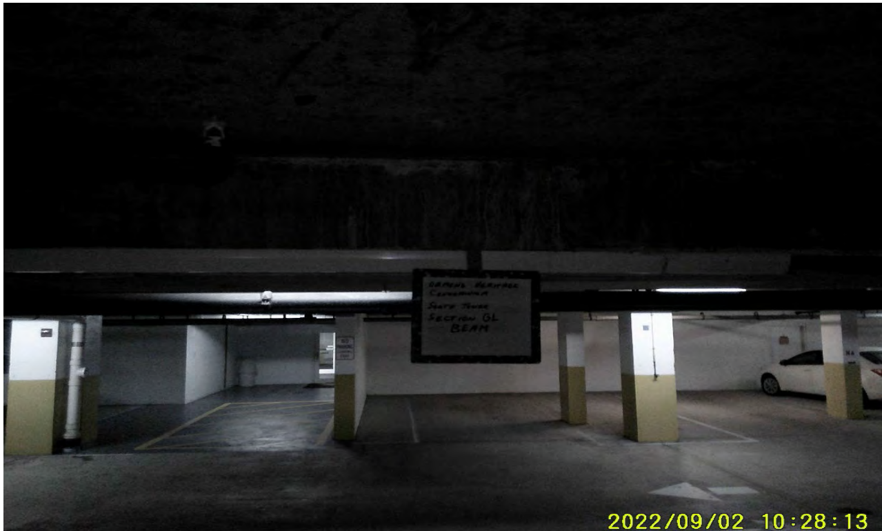
Photograph 25: South Tower, Parking Garage Section GL
