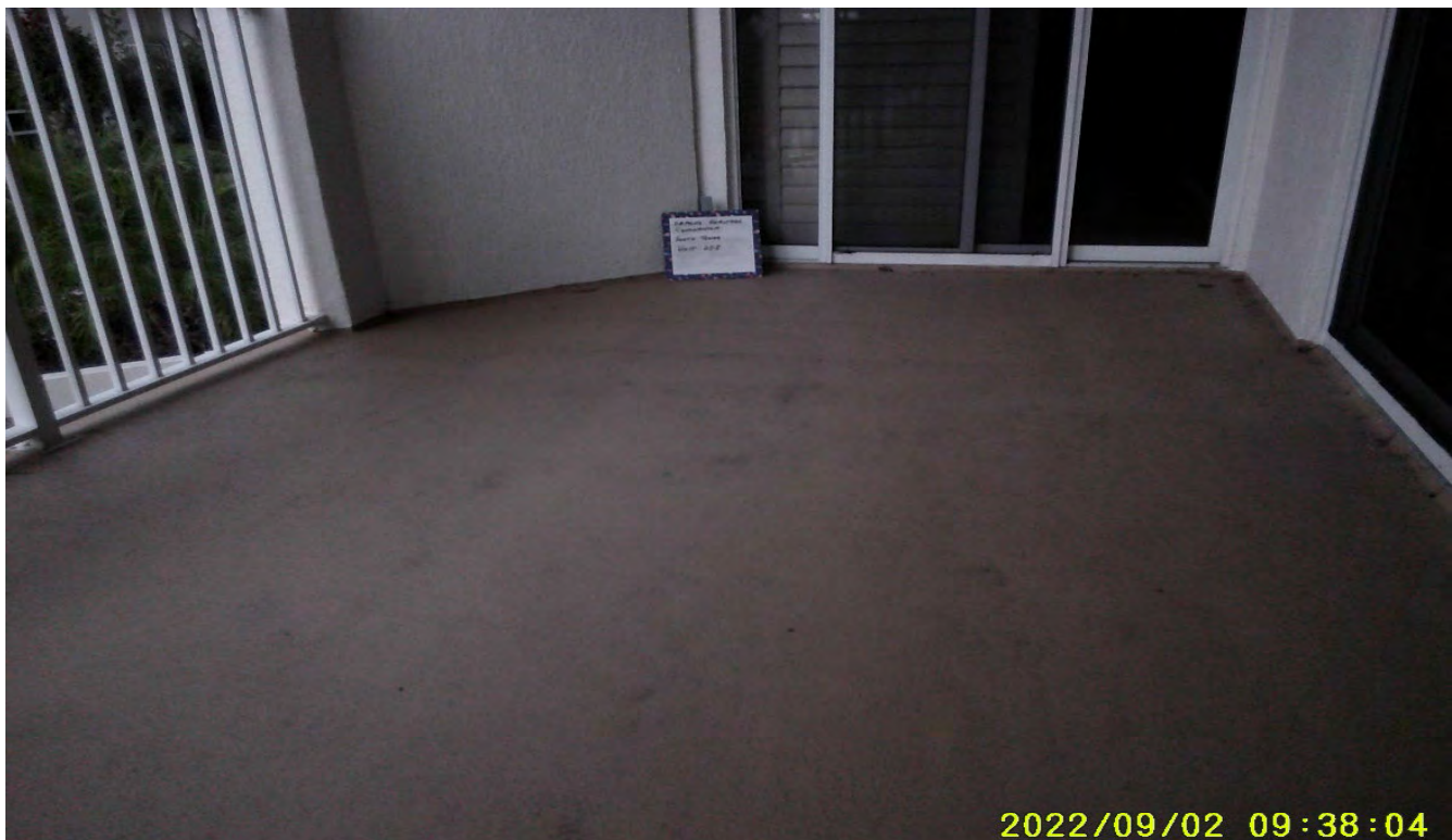
Photograph 38: Balcony (Misc. Location)
