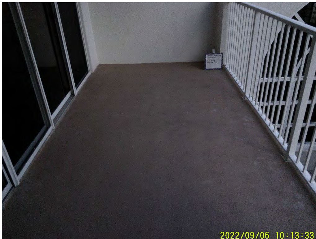
Photograph 94: Balcony (Misc. Location)
