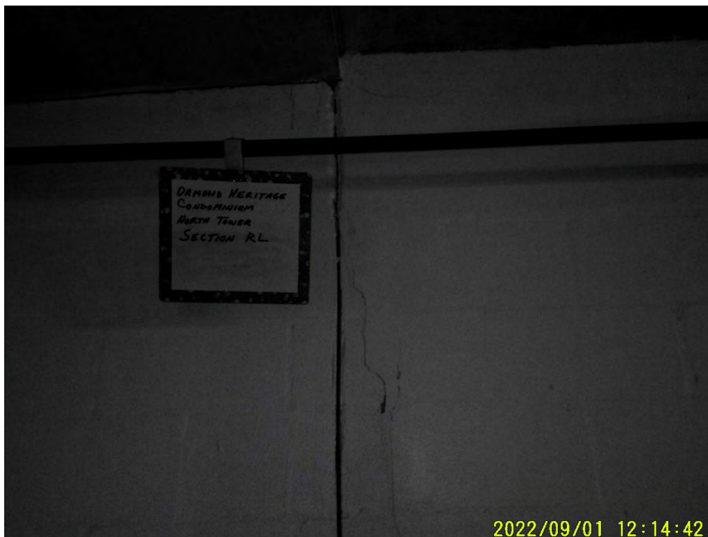
Photograph 71: North Tower, Parking Garage Section RL
