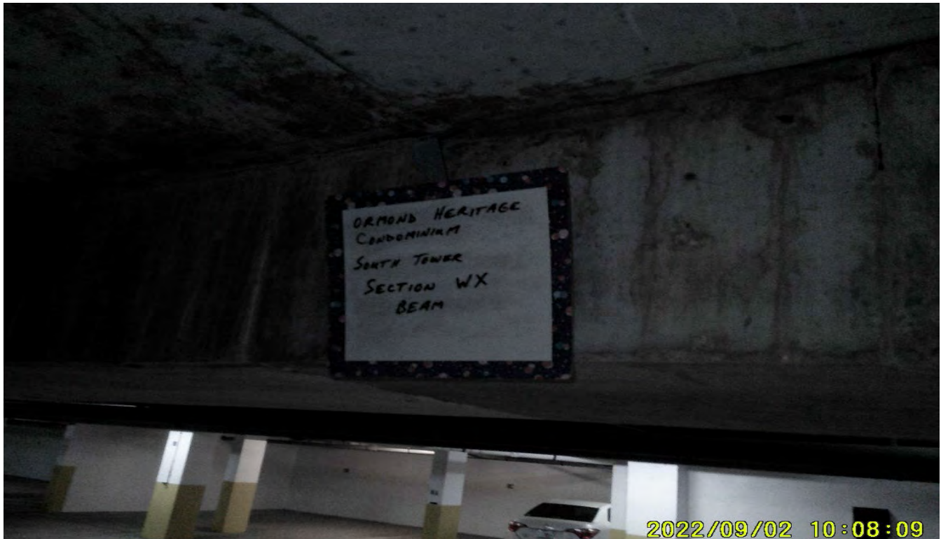
Photograph 31: South Tower, Parking Garage Section WX
