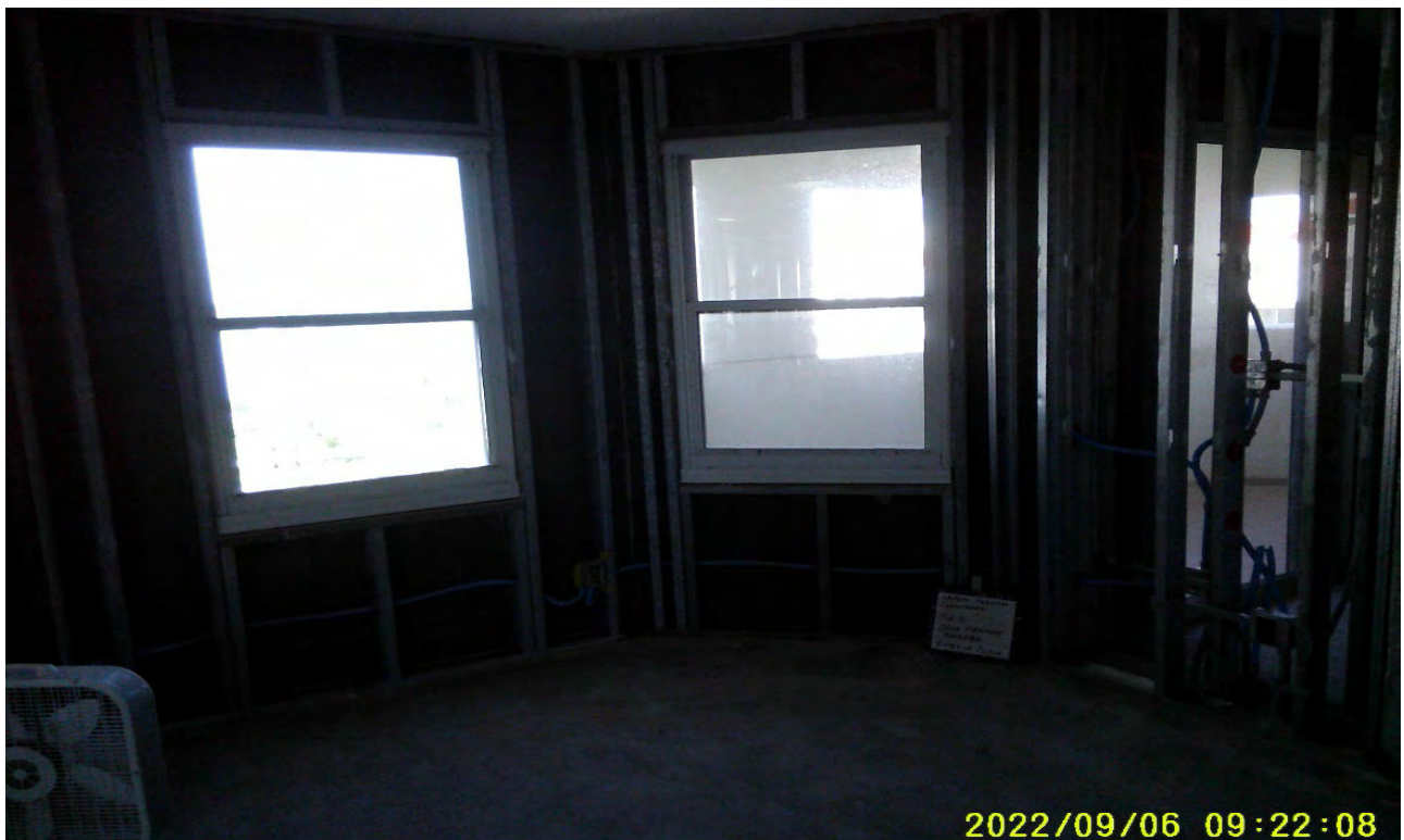
Photograph 8: Phase 2 Open Framing, Ext. Plane
