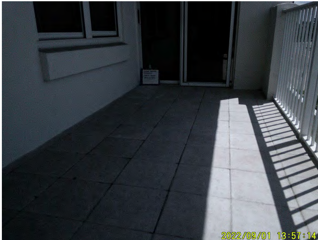
Photograph 55: Balcony (Misc. Location)
