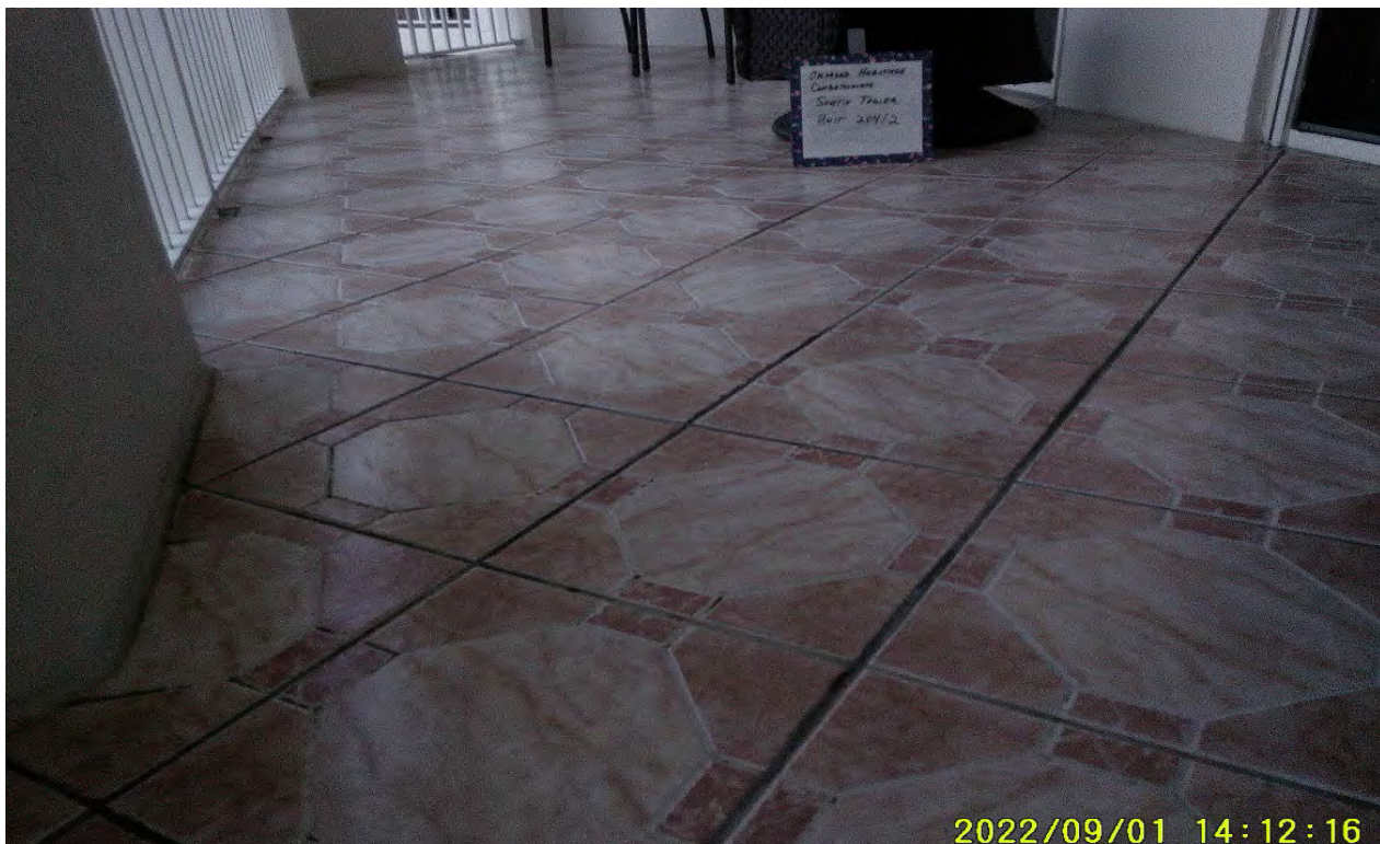
Photograph 52: Balcony, South Tower Unit 204/2
