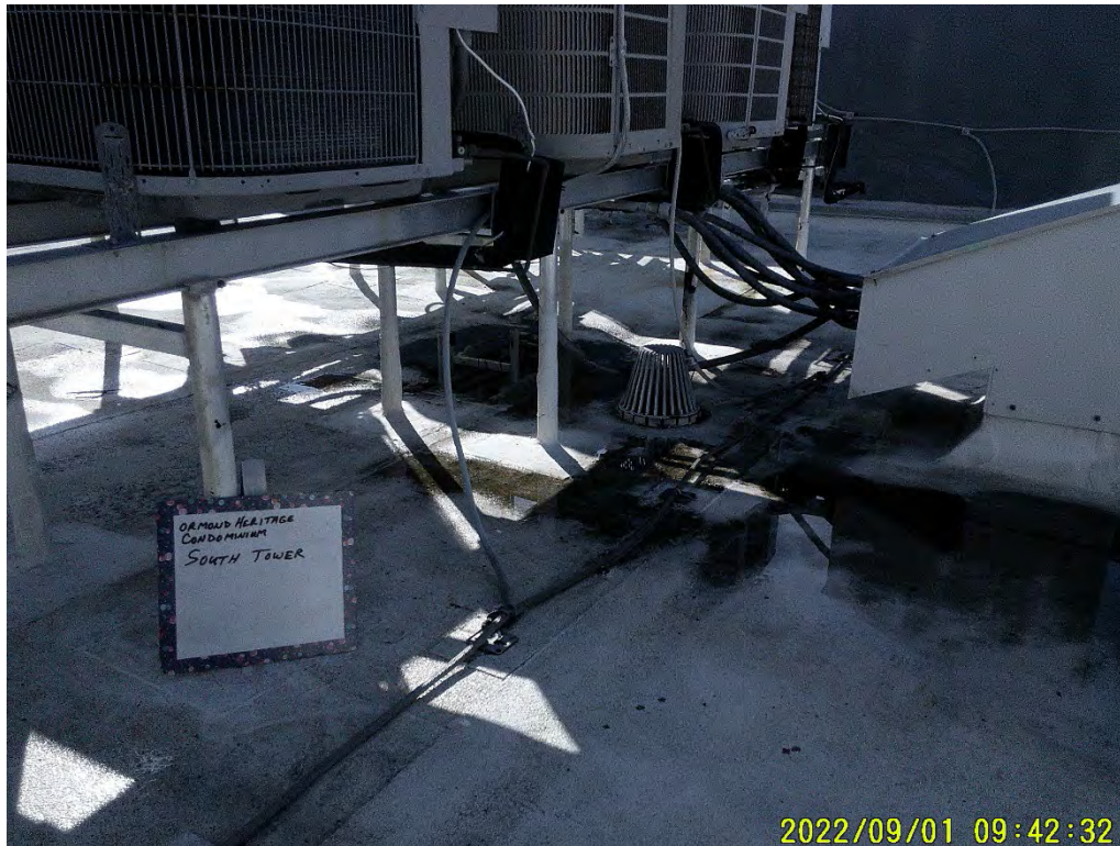
Photograph 101: South Tower, Roof
