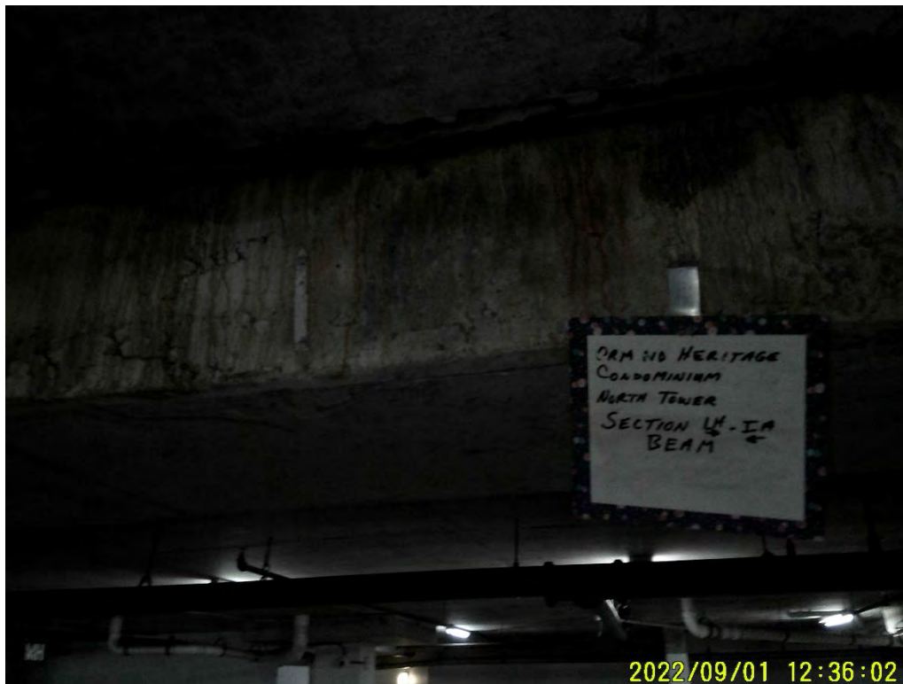
Photograph 65: North Tower, Parking Garage Section LH-IA
