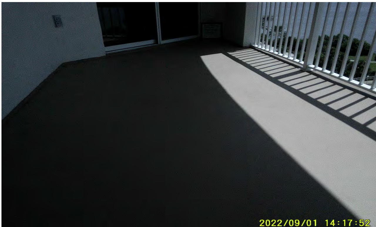
Photograph 50: Balcony South Tower – Phase 4/1, 4/2, and 4/3
