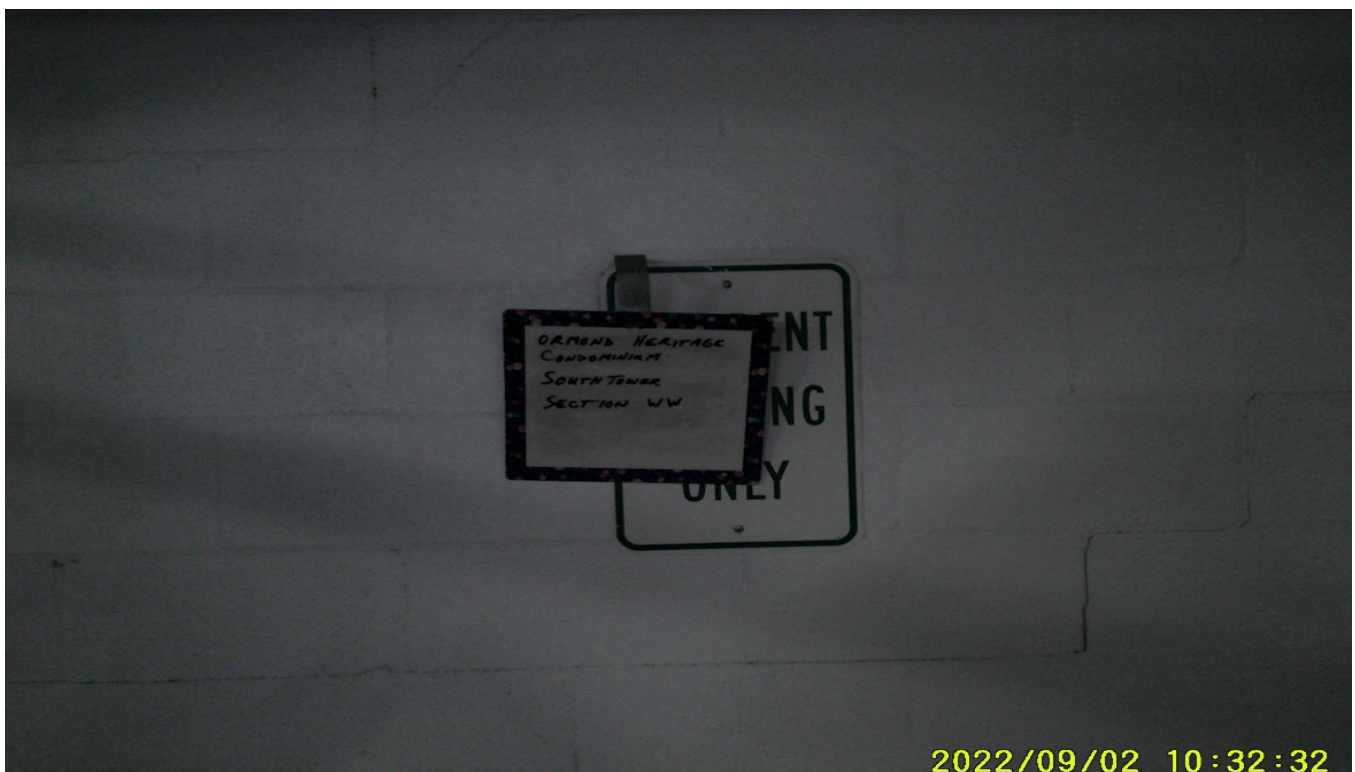
Photograph 24: South Tower, Parking Garage Section WW
