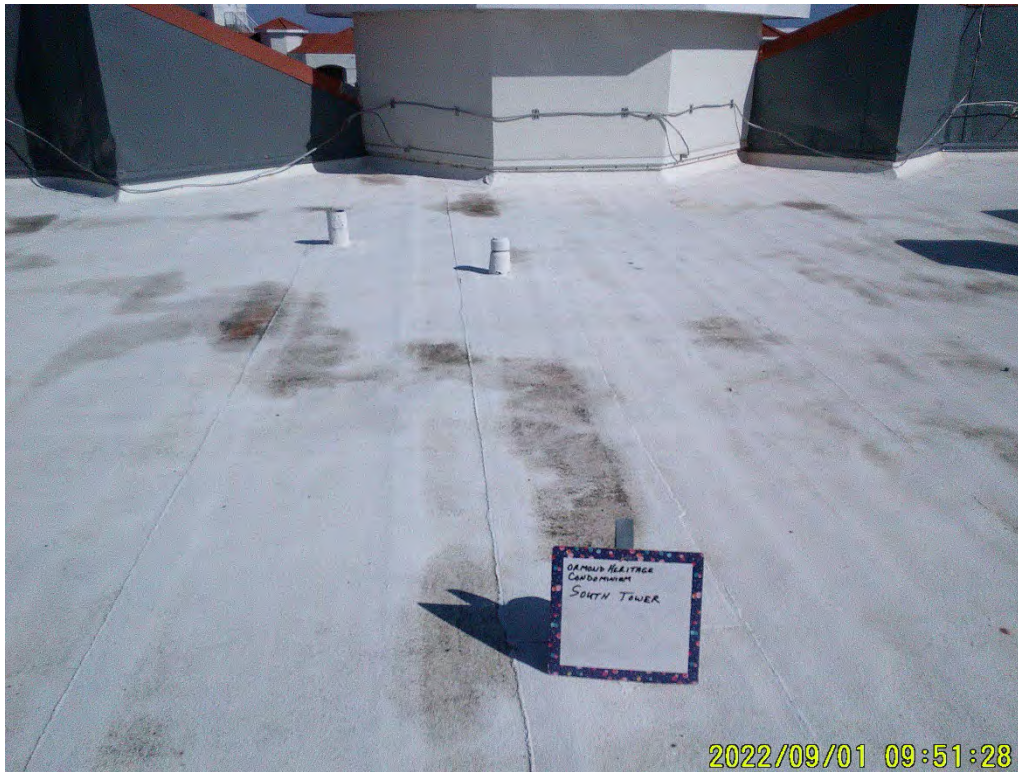
Photograph 89: South Tower, Roof
