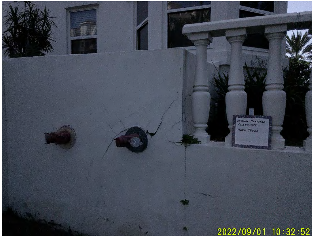
Photograph 83: Façade South Wall Tower
