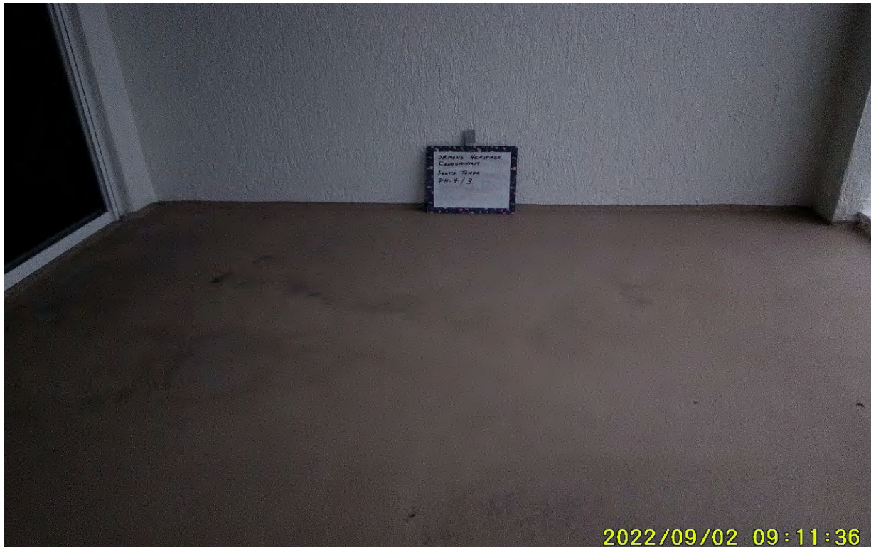
Photograph 47: Balcony South Tower – Phase 4/1, 4/2, and 4/3
