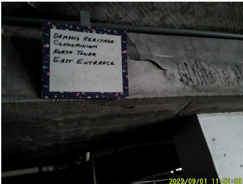
Photograph 74: North Tower Parking Garage East Entrance
