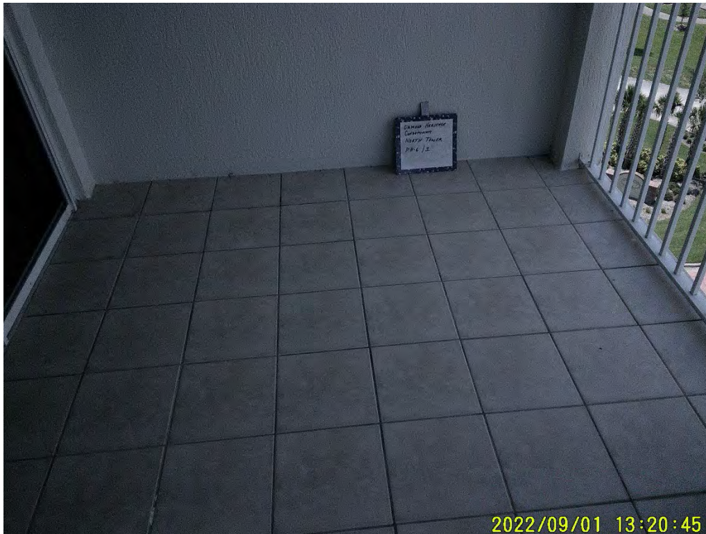
Photograph 61: Balcony, North Tower – Phase 6/1
