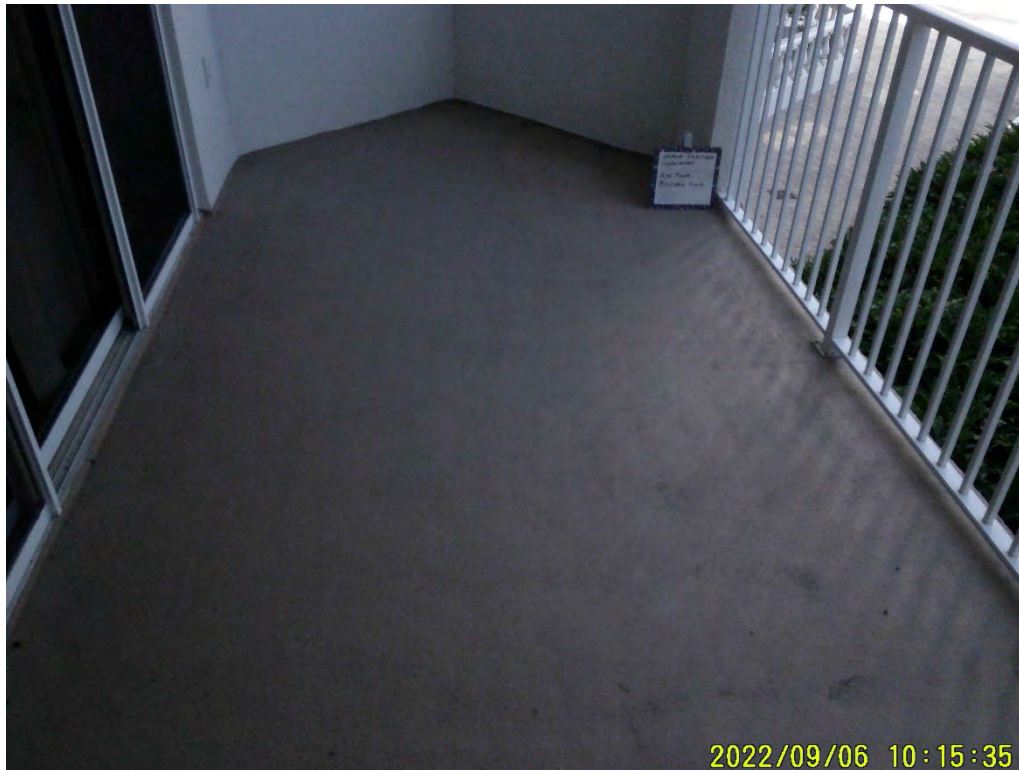
Photograph 93: Balcony (Misc. Location)
