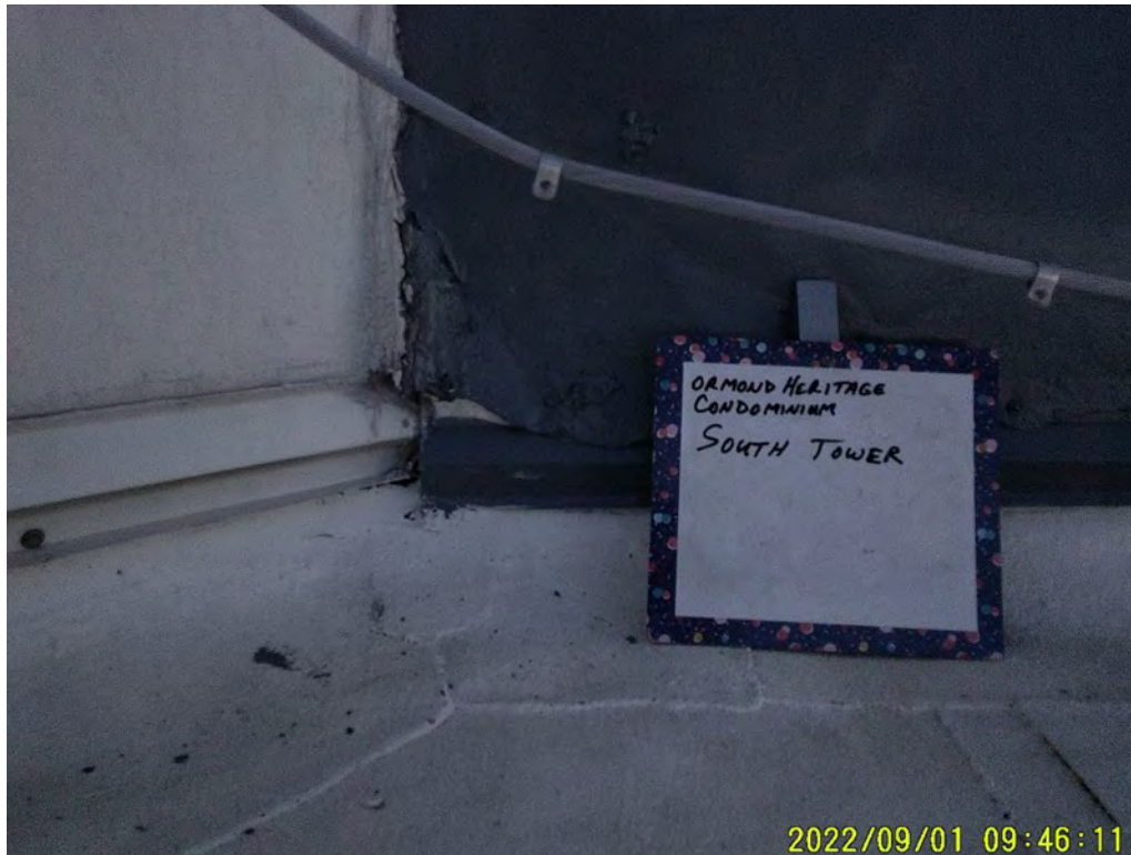
Photograph 91: South Tower, Roof
