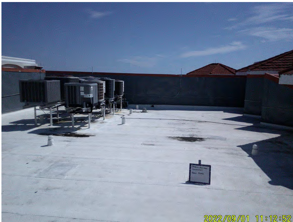
Photograph 76: North Tower, Roof
