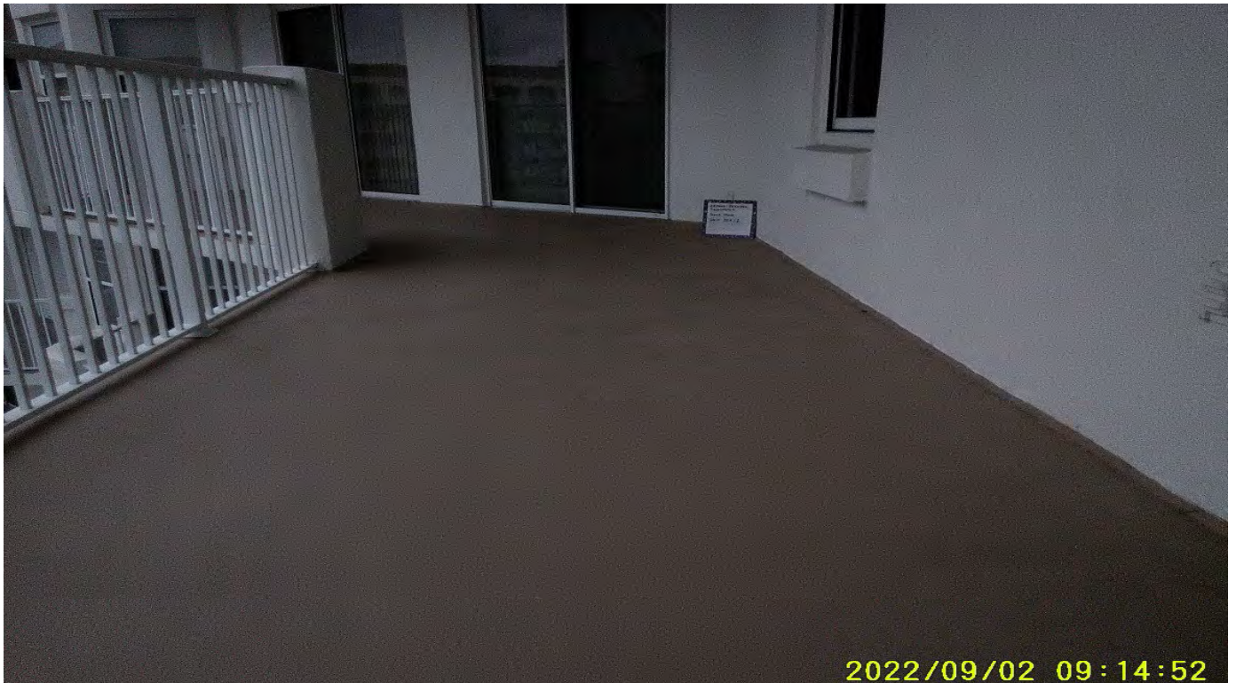
Photograph 45: Balcony (Misc. Location)
