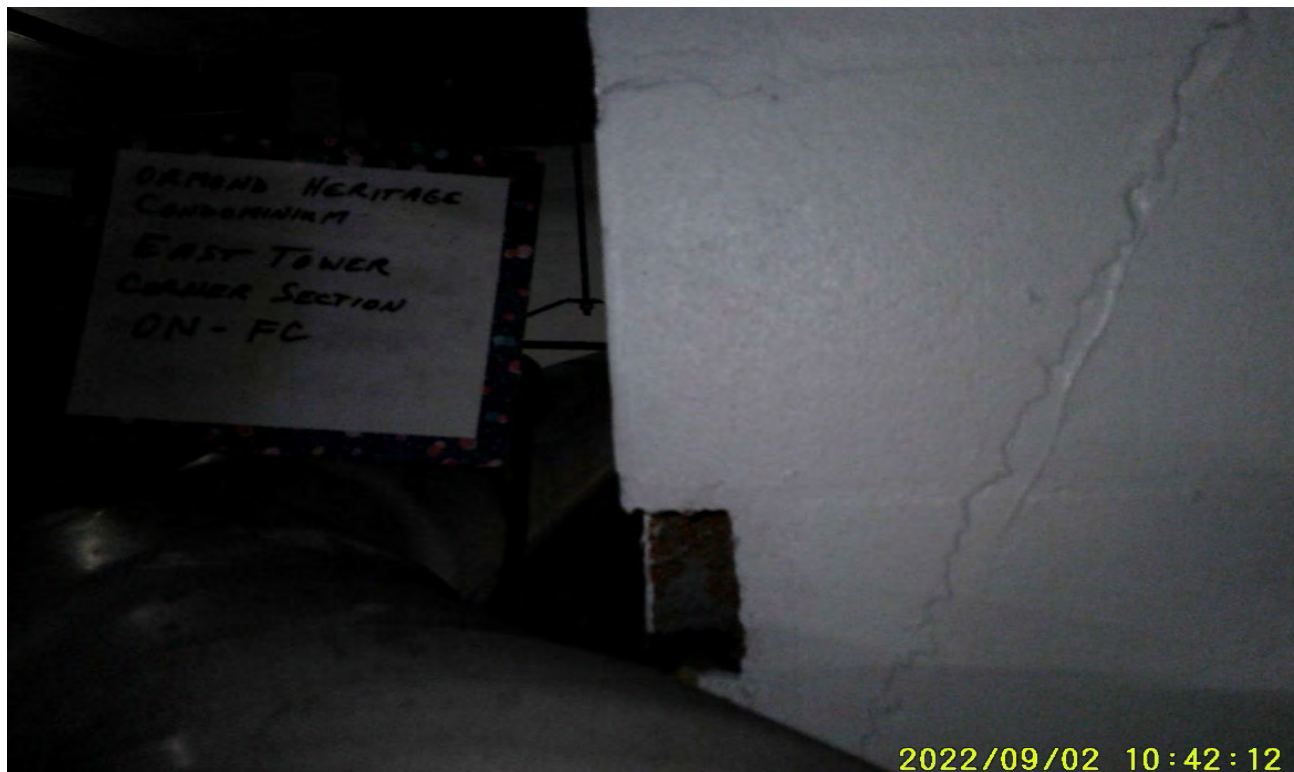
Photograph 21: East Tower, Parking Garage Section FC
