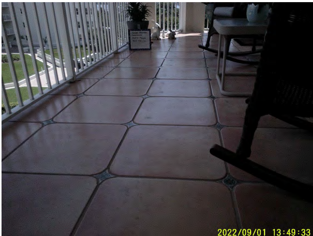
Photograph 58: Balcony (Misc. Location)
