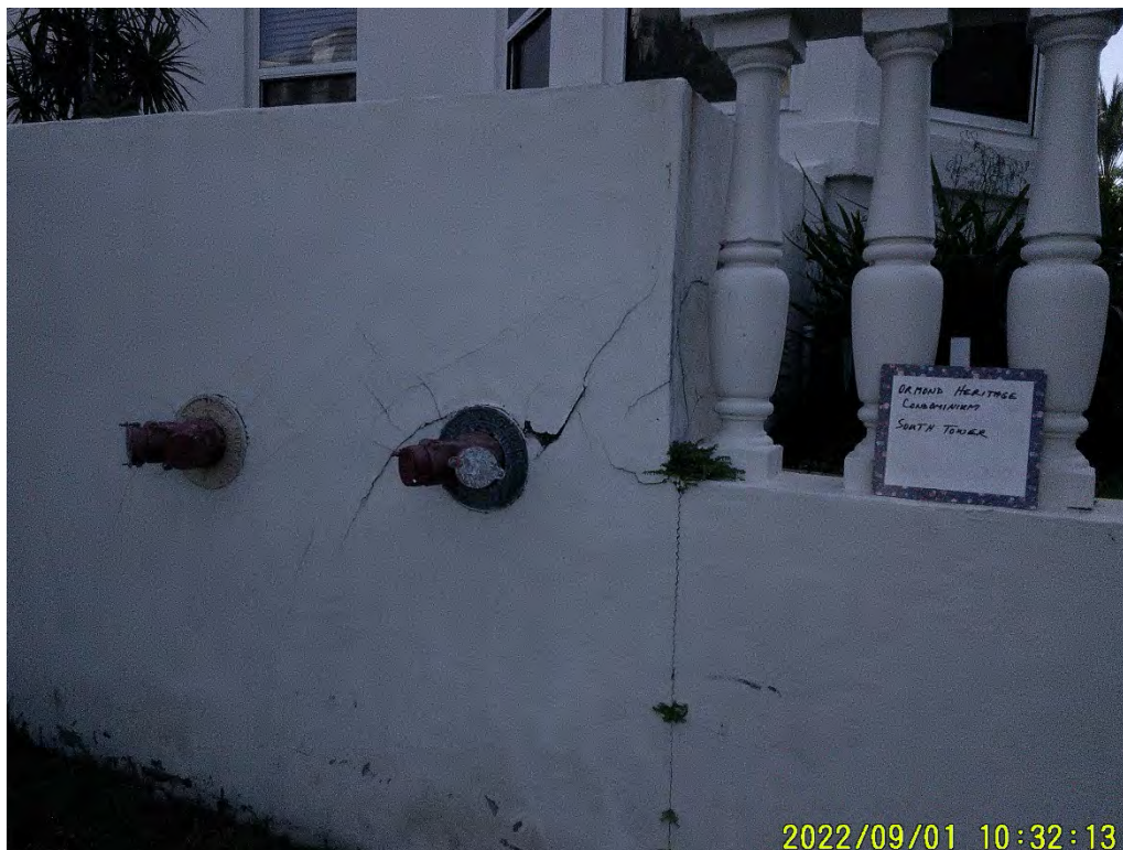
Photograph 84: Façade South Wall Tower
