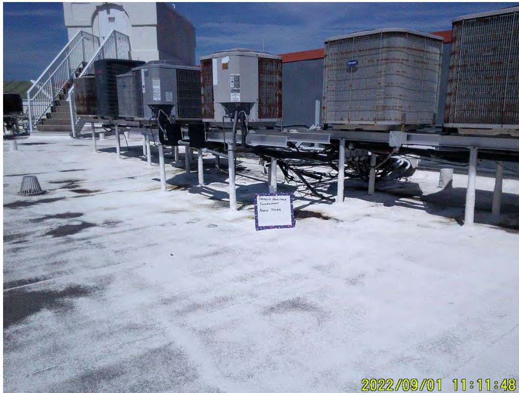
Photograph 77: North Tower, Roof
