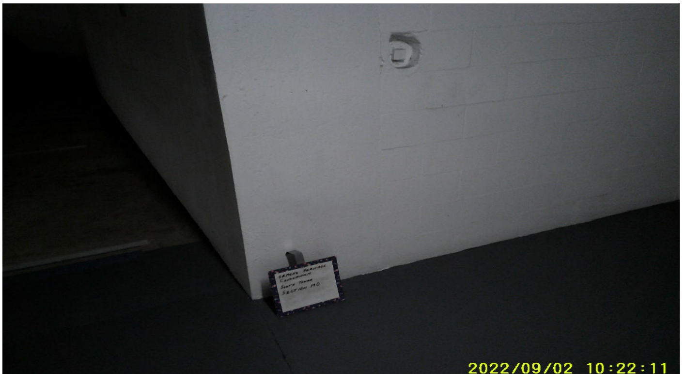
Photograph 28: South Tower, Parking Garage Section MO
