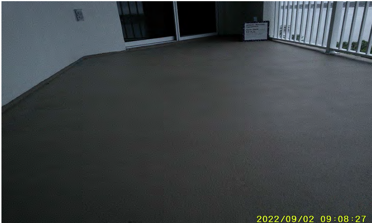
Photograph 49: Balcony South Tower – Phase 4/1, 4/2, and 4/3
