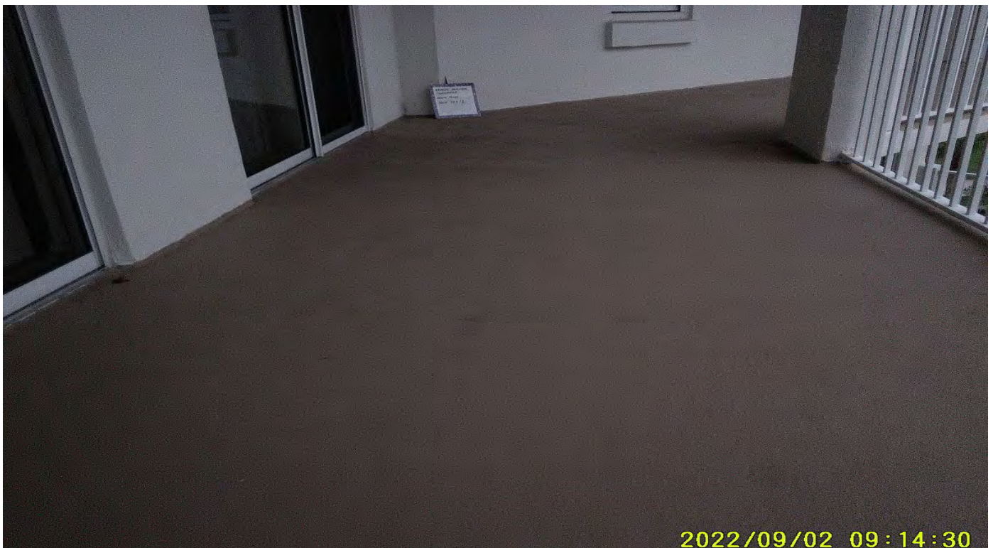
Photograph 46: Balcony (Misc. Location)
