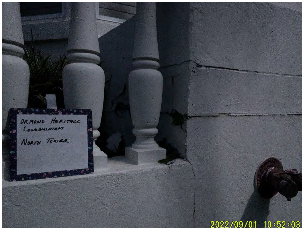
Photograph 82: Façade North Tower
