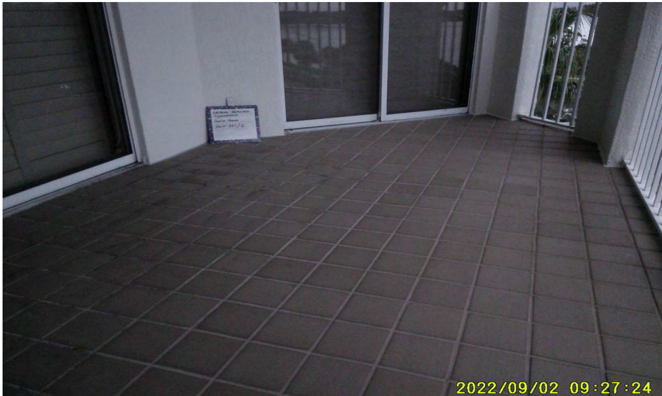
Photograph 41: Balcony (Misc. Location)
