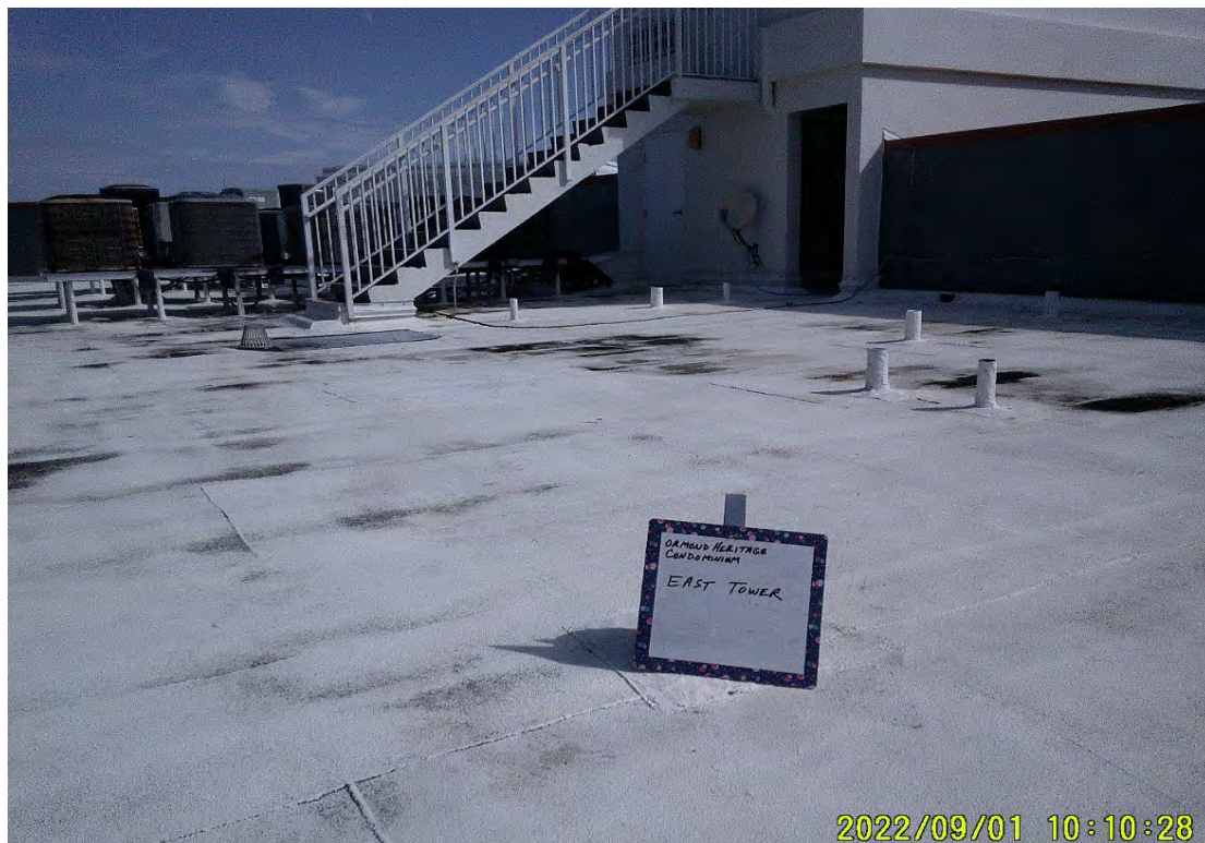
Photograph 88: East Tower, Roof
