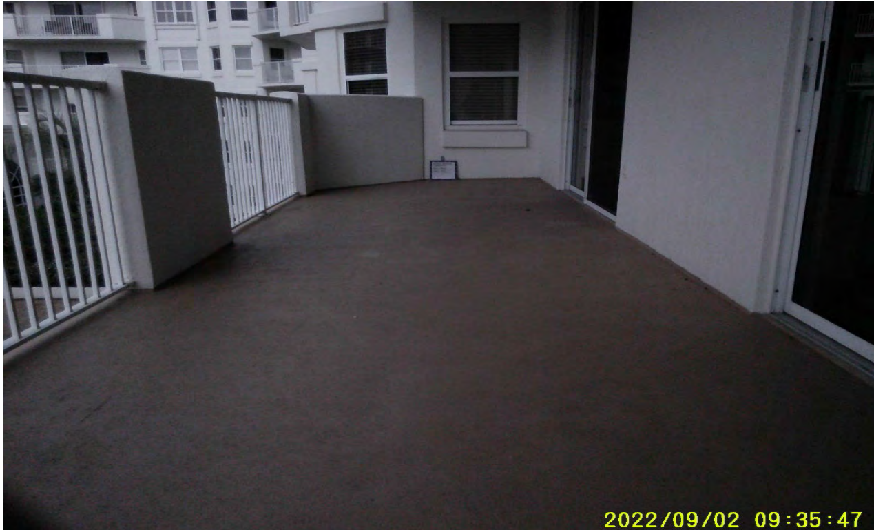
Photograph 39: Balcony (Misc. Location)
