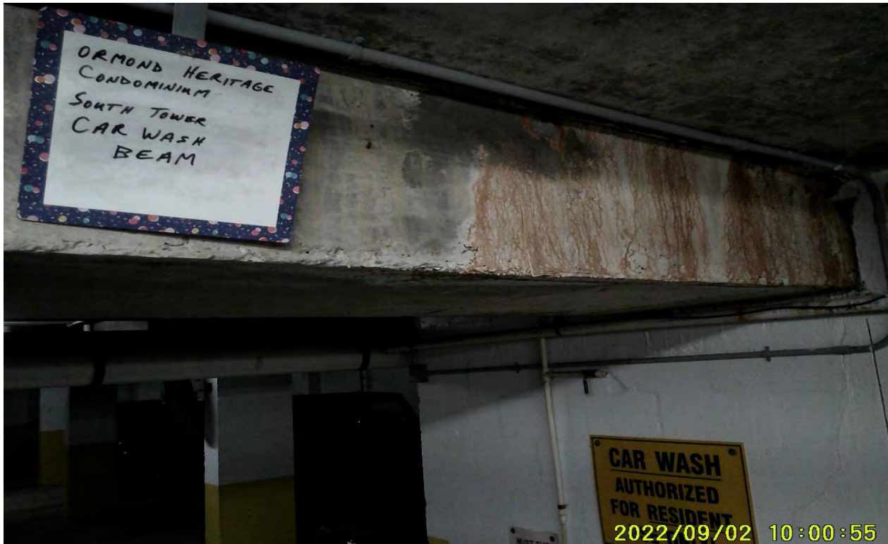
Photograph 37: South Tower, Parking Garage Car Wash
