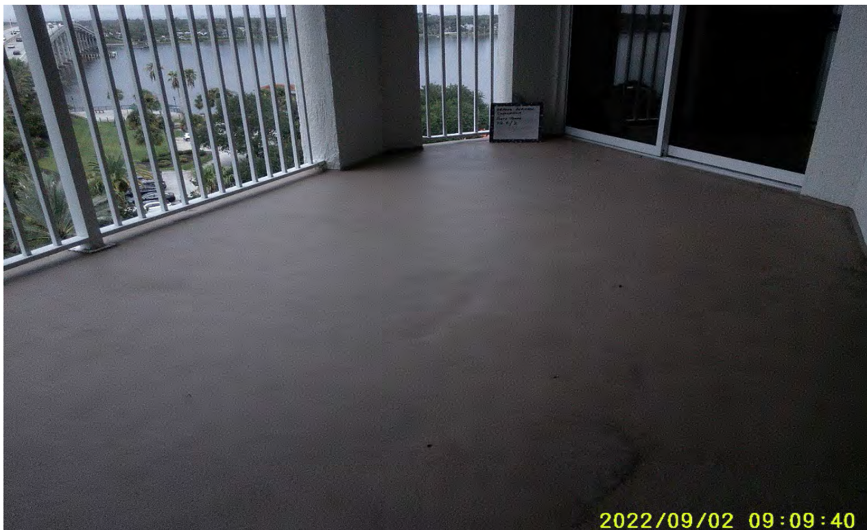
Photograph 48: Balcony South Tower – Phase 4/1, 4/2, and 4/3
