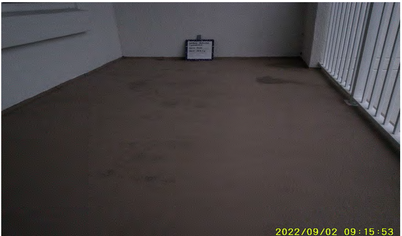
Photograph 44: Balcony (Misc. Location)
