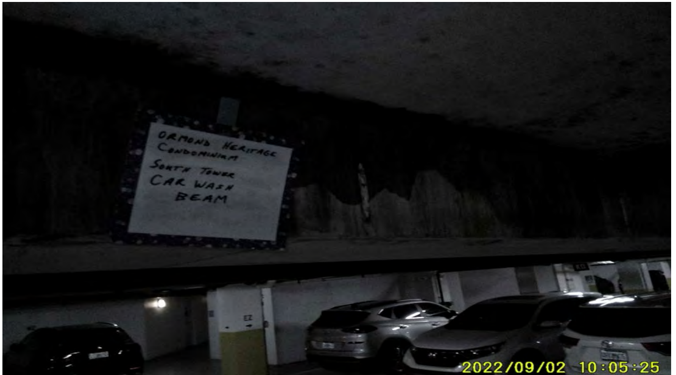
Photograph 33: South Tower, Parking Garage Car Wash
