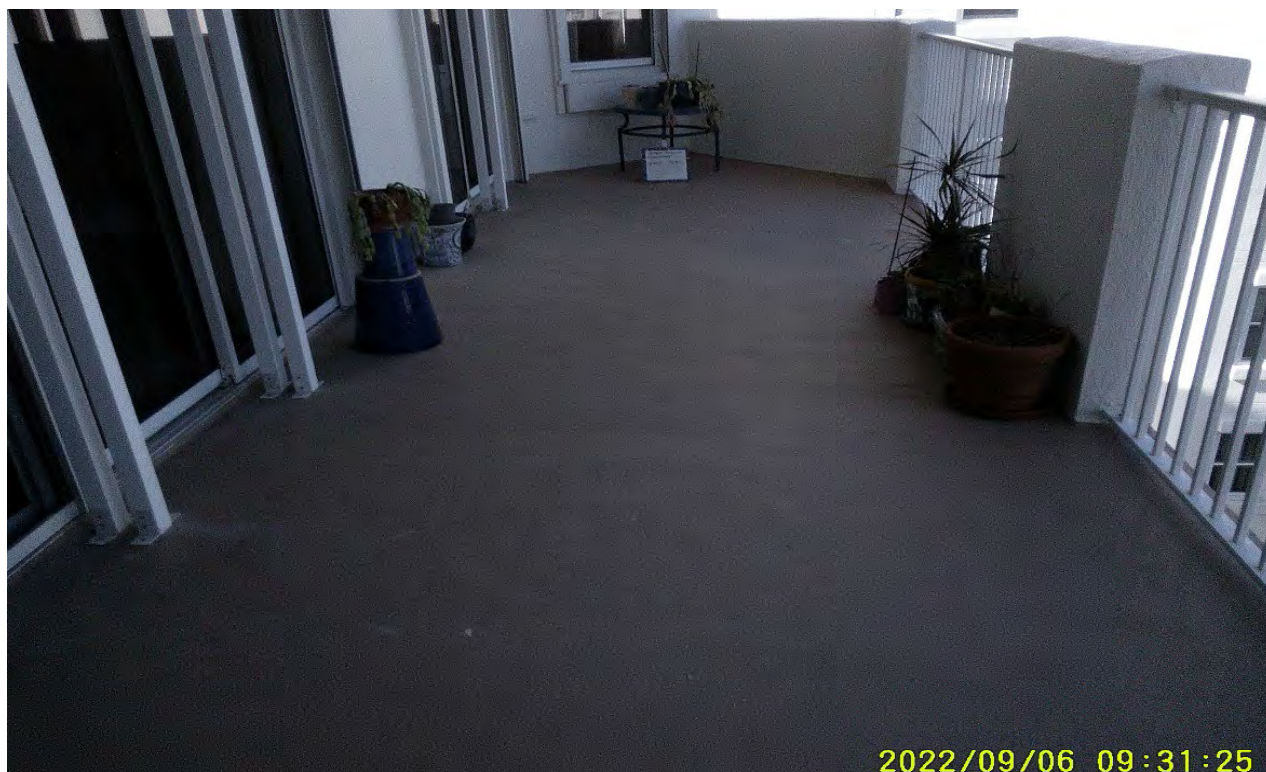
Photograph 3: Balcony (Misc. Location)
