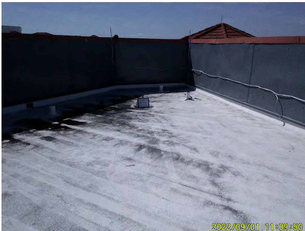
Photograph 80: North Tower, Roof
