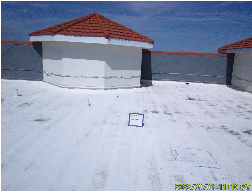
Photograph 79: North Tower, Roof
