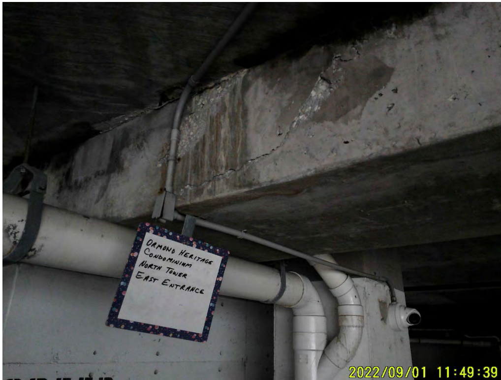
Photograph 75: North Tower Parking Garage East Entrance
