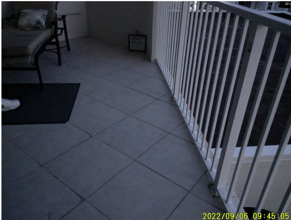
Photograph 99: Balcony (Misc. Location)
