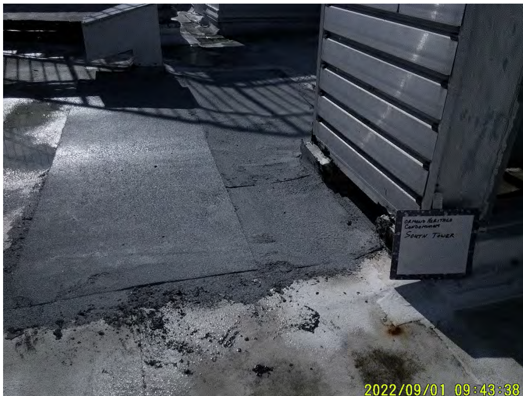
Photograph 92: South Tower, Roof
