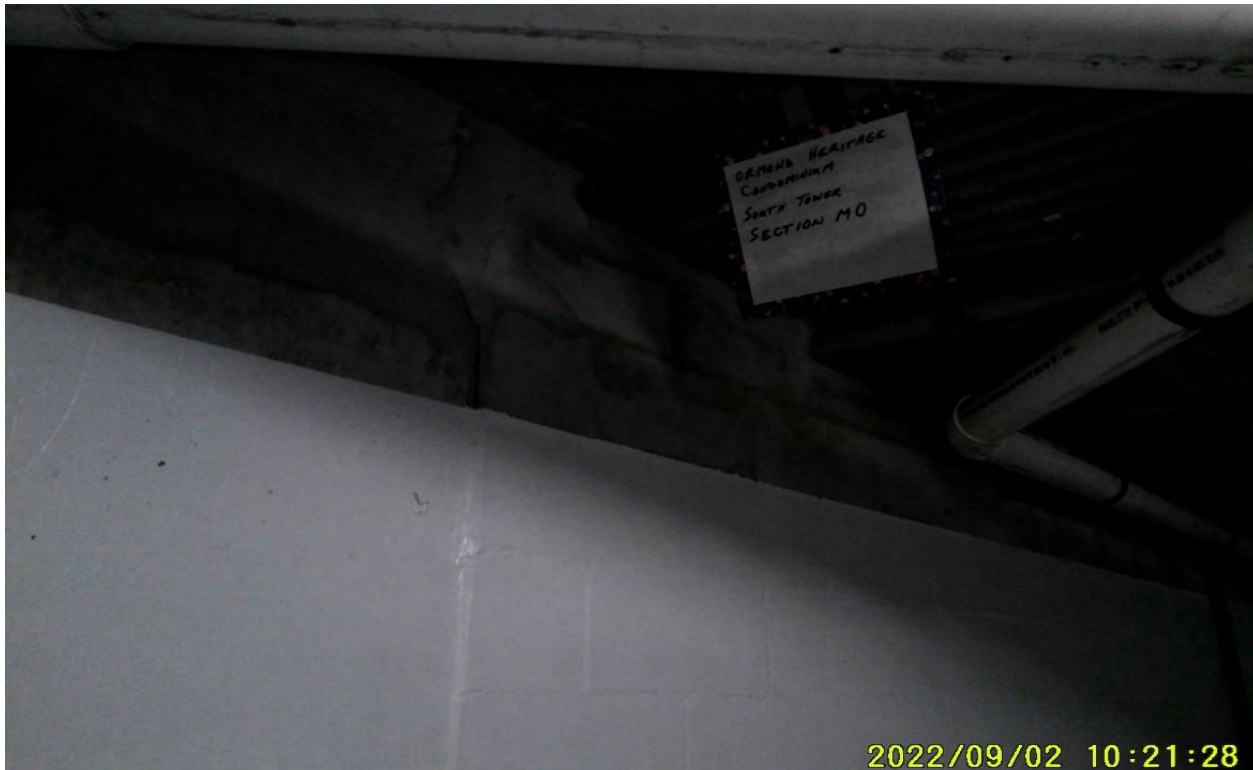
Photograph 27: South Tower, Parking Garage Section MO
