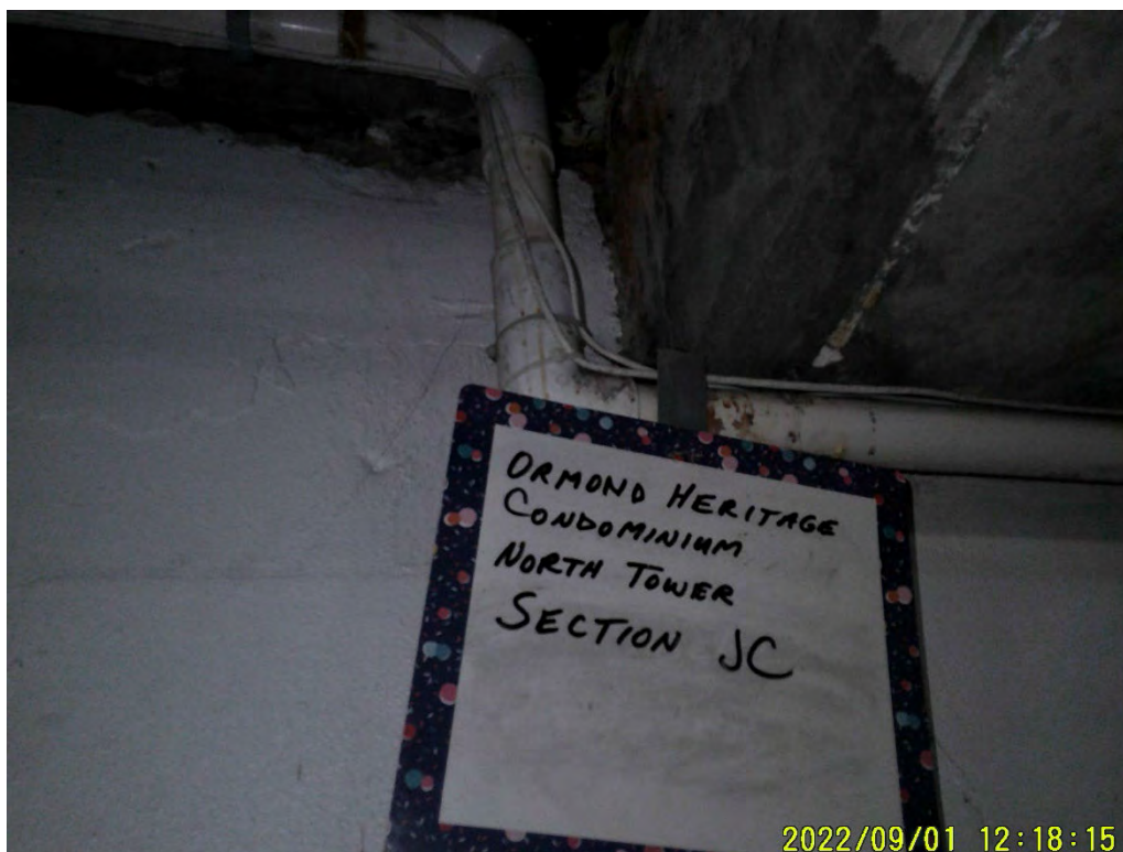
Photograph 70: North Tower, Parking Garage Section JC
