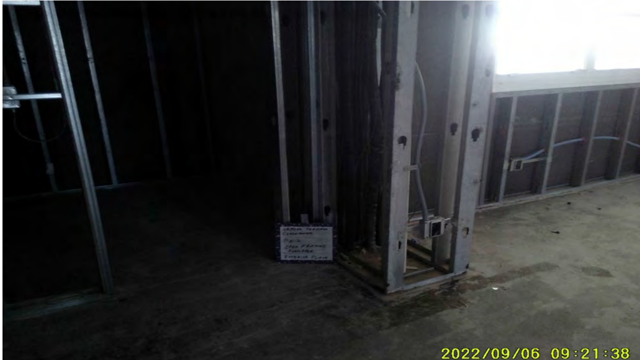
Photograph 9: Phase 2 – Open Framing, Ext. Plane
