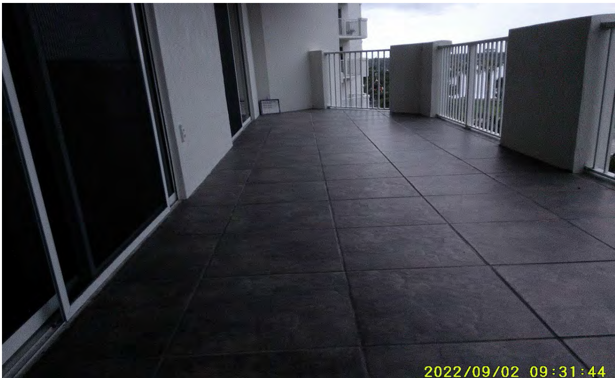
Photograph 40: Balcony (Misc. Location)
