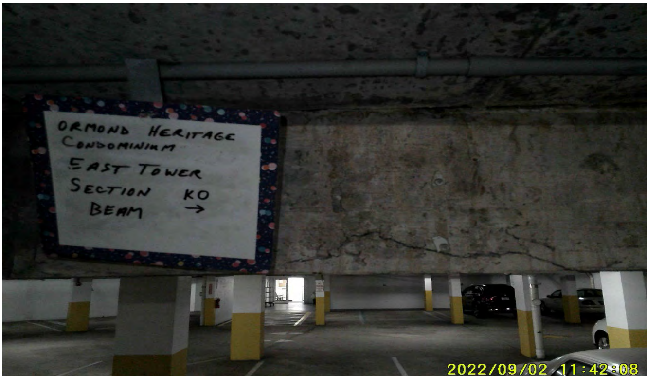
Photograph 14: East Tower, Parking Garage Section KO
