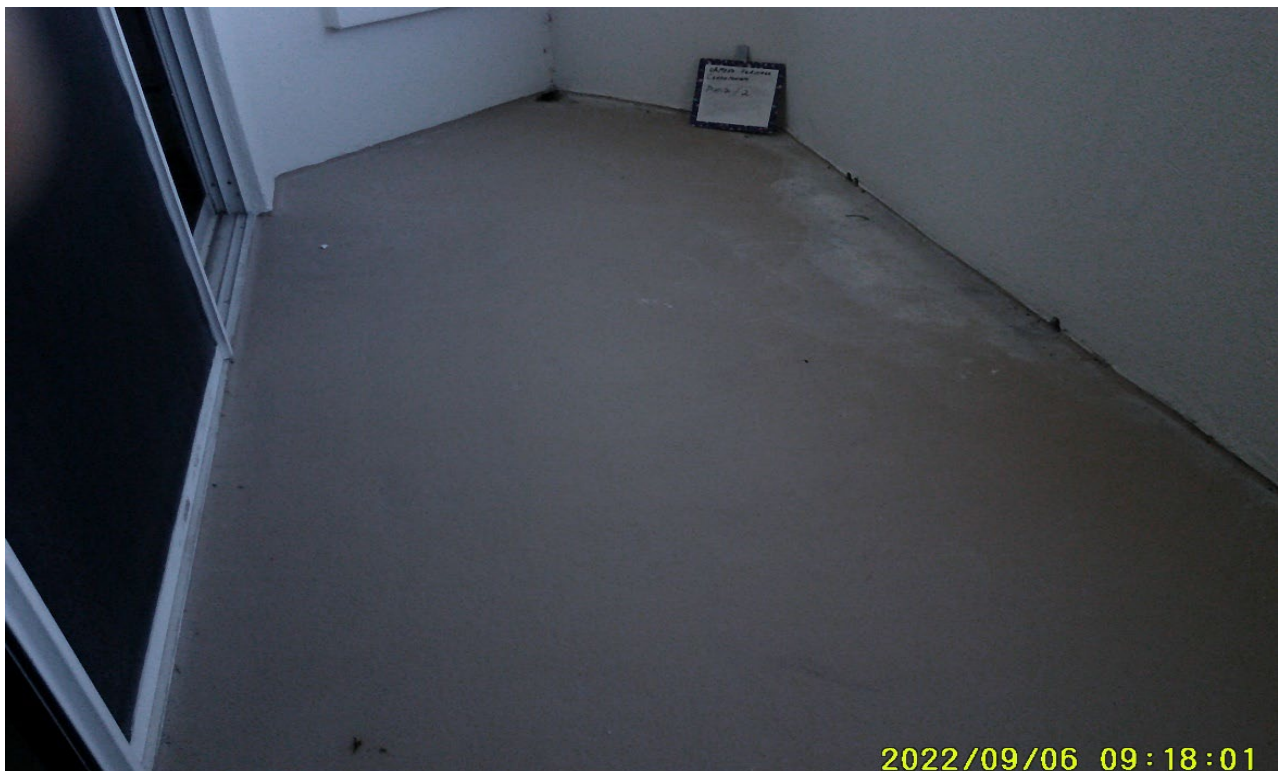
Photograph 10: Balcony (Misc. Location)
