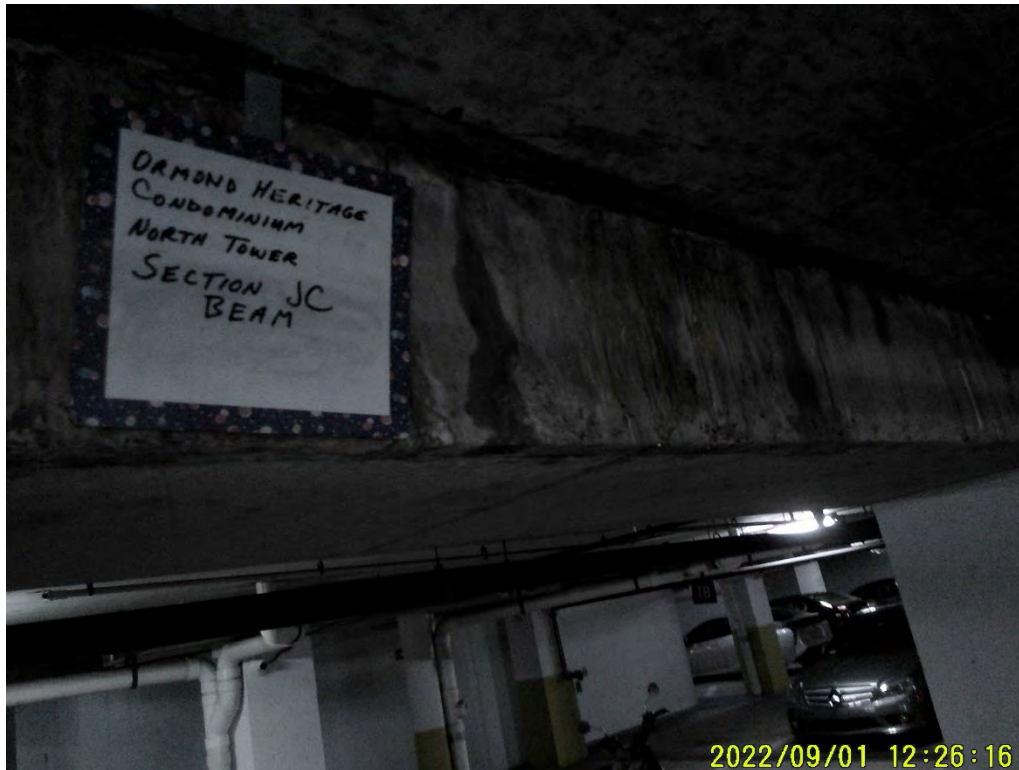
Photograph 67: North Tower, Parking Garage Section JC
