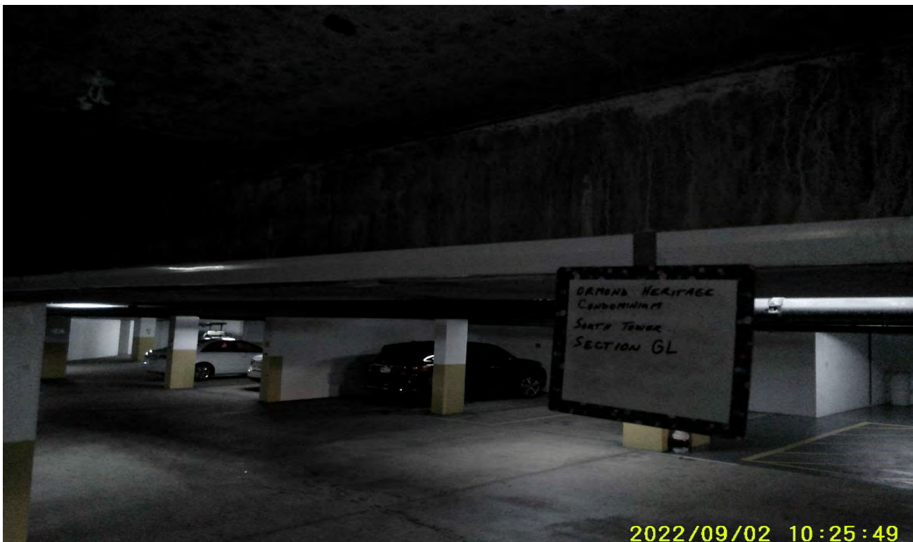
Photograph 26: South Tower, Parking Garage Section GL
