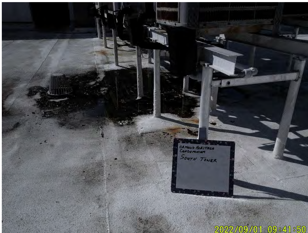
Photograph 102: South Tower, Roof
