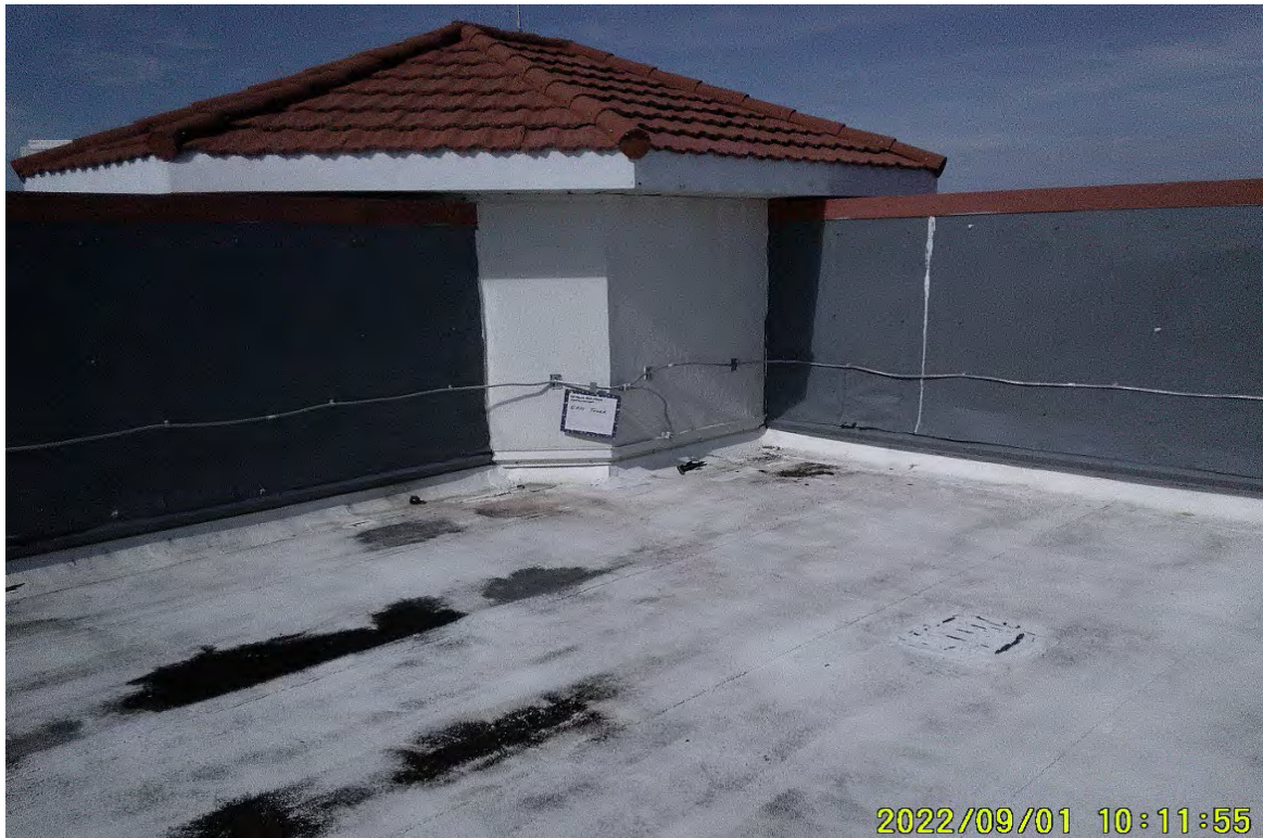
Photograph 87: East Tower, Roof
