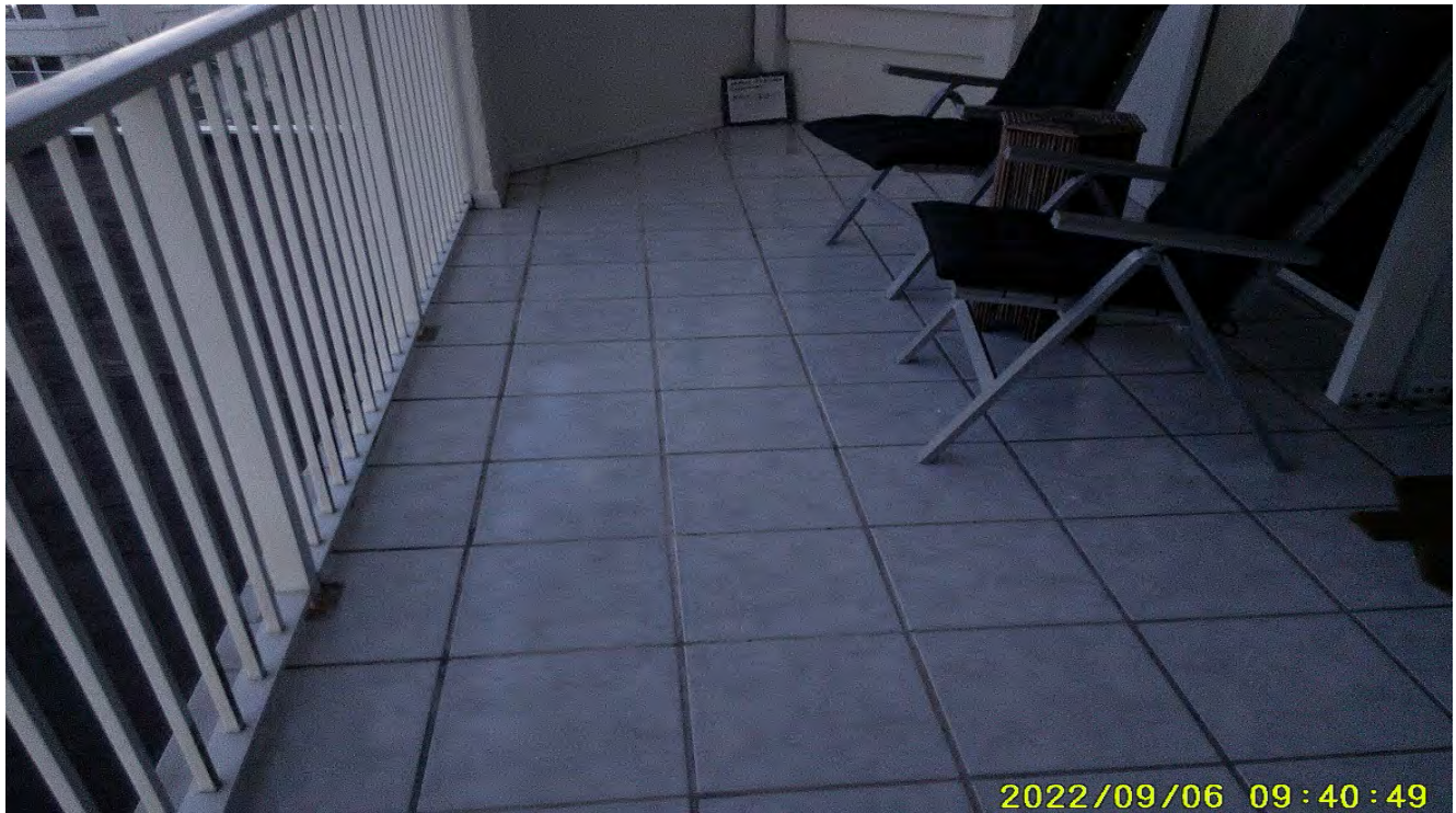
Photograph 1: Balcony (Misc. Location)
