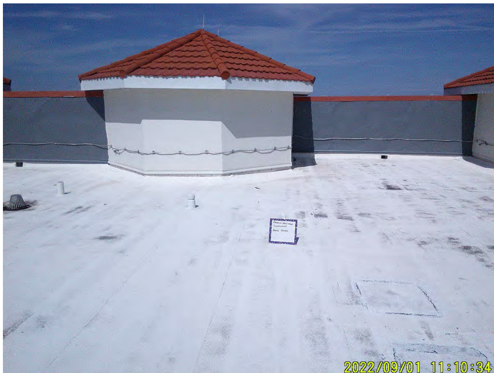
Photograph 78: North Tower, Roof
