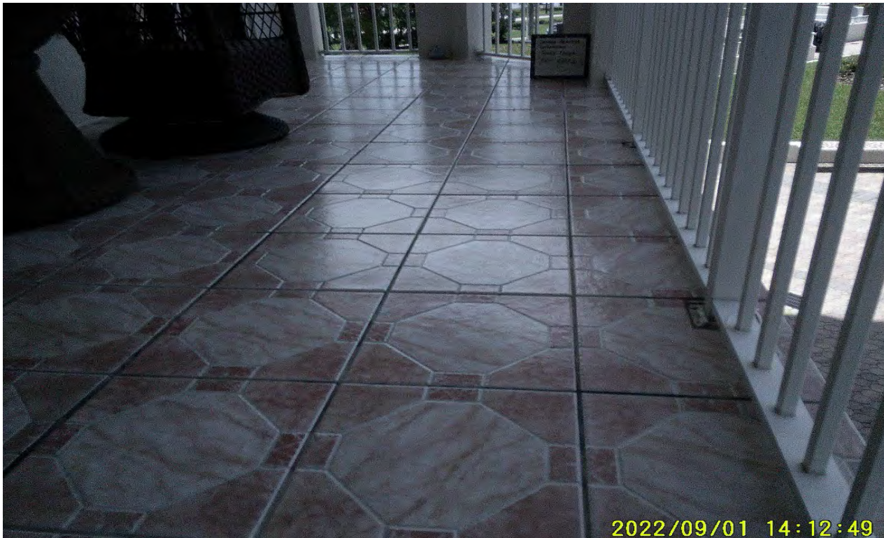
Photograph 51: Balcony, South Tower Unit 204/2
