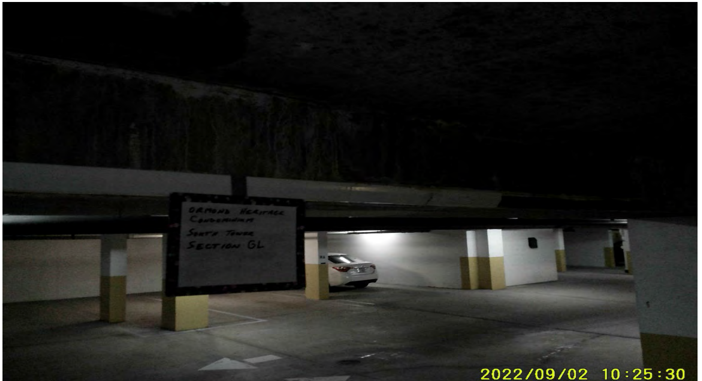
Photograph 27: South Tower, Parking Garage Section GL
