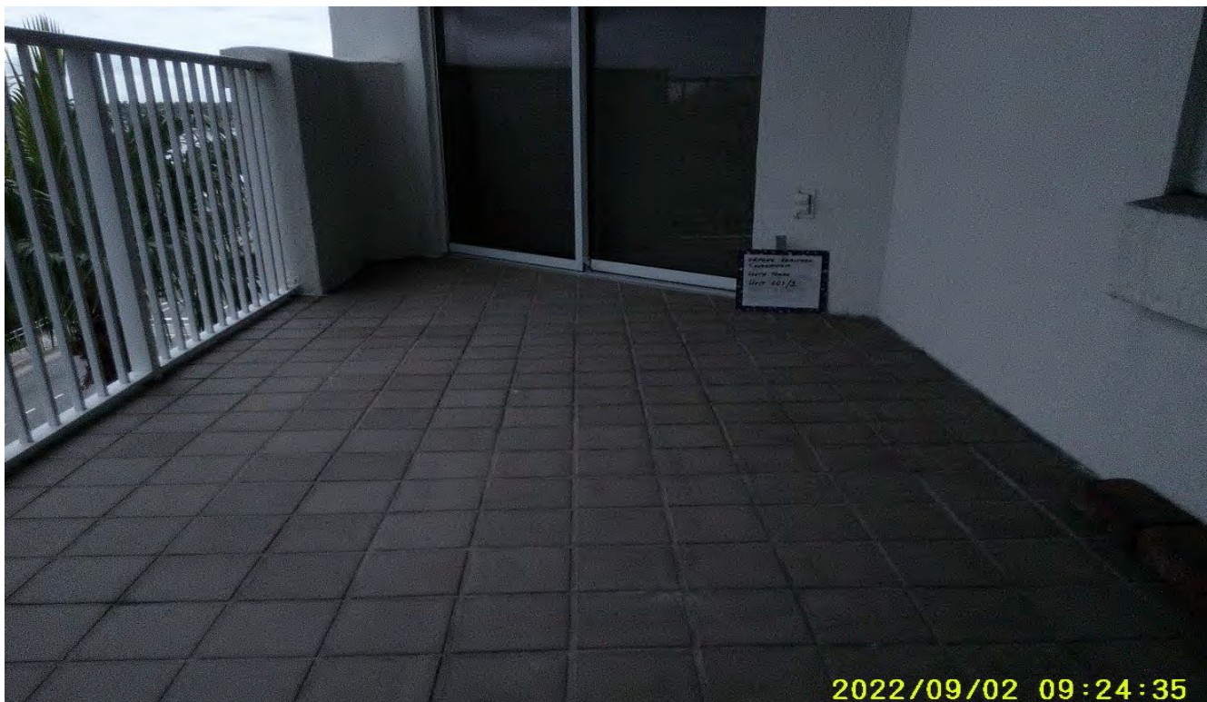
Photograph 42: Balcony (Misc. Location)
